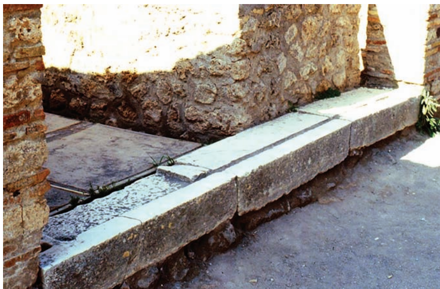
FIGURE 15.5. Groove for a barricade to a shop entrance for closing up at night. (Photo by Glenn Storey)
