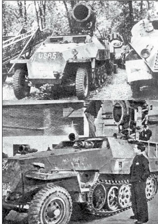
The Uhu system on a half-track reconnaissance vehicle. (Photo: CIOS)
