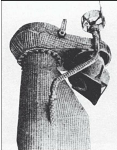
The snorkel of a Type XXI submarine, covered in “stealth” material. (Photo from the author's collection)
